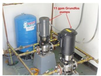
downstream complies with the regulatory requirements for safe drinking water. A blueprint of a booster station with a single pump configuration can be seen at <u>(Appendix VI – T2)</u>.
