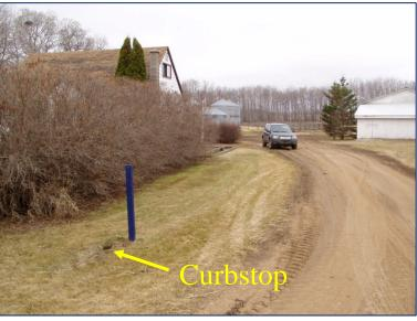
consistent, locating it during an emergency will be quicker, less stressful and may help to avoid further damages to equipment and property. Routine maintenance should also be quicker and easier if curbstops are easily identified and can be cross referenced with corresponding drawings to verify valve placement.
