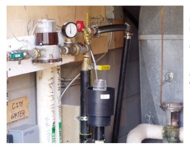
Sample ports or stations should be set up at pumphouses and booster stations to monitor water quality. Data should be recorded and evaluated as determined in your Permit to Operate. It is strongly recommended that operators have a safe and user- friendly place to draw samples for analysis.
