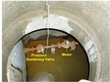
Depending on the source of the water supply, a below ground metering vault or "manhole" may be required. If the source water is part of an existing pipeline and infrastructure. the manhole connections are often used as a starting point for the distribution system. The manhole generally includes a water meter, isolation valve, backflow prevention device, and in some cases, a pressure sustaining valve. The manhole and connection may be installed by the source utility (i.e. City of
