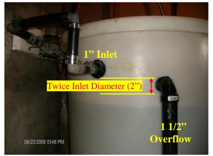
An air gap device is a relativelv inexpensive device that is created in the subscriber's cistern or storage tank and if configured correctly, has a verv high degree of backflow prevention. An air gap is achieved by ensuring that the elevation of the lowest point of the inlet or point where water discharged into the is storage tank is above the lip of the overflow. This means that if the float assembly in the storage
