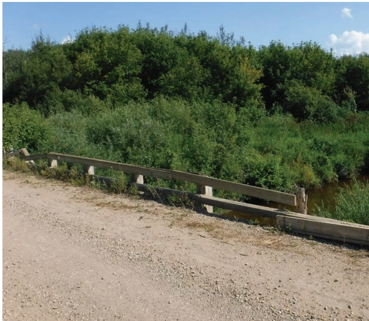
The images on pages 18 and 19 depict typical damage to bridge safety components in RMs across the province. Far left: broken post on a hazard size (abutment 2 left hand side). Above (clockwise, left to right): severe wear on hazard size coating (abutment 2 right hand side hazard sign); downed hazard sign; and a missing and broken left hand side rail.
