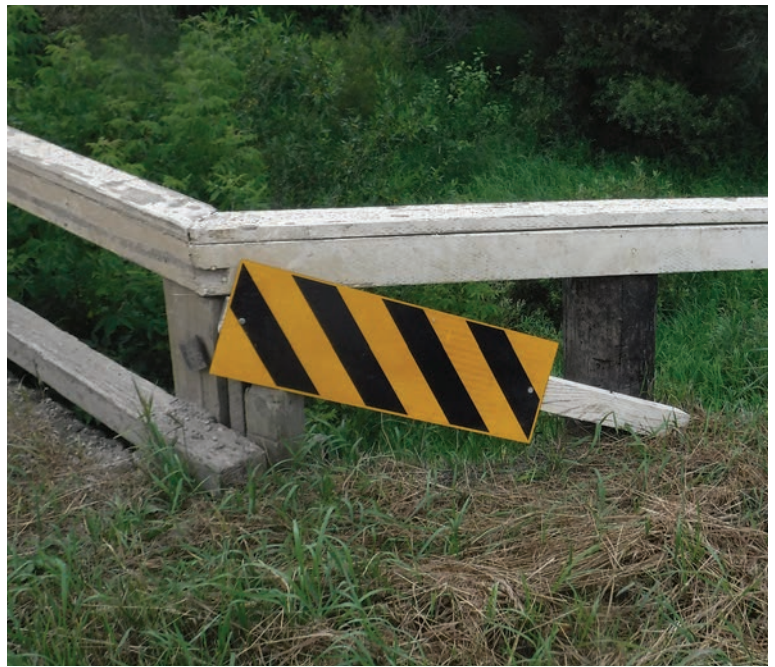
The images on pages 18 and 19 depict typical damage to bridge safety components in RMs across the province. Far left: broken post on a hazard size (abutment 2 left hand side). Above (clockwise, left to right): severe wear on hazard size coating (abutment 2 right hand side hazard sign); downed hazard sign; and a missing and broken left hand side rail.
