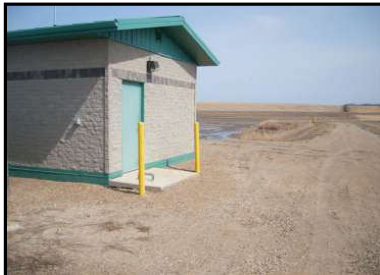
Well and Pump House
